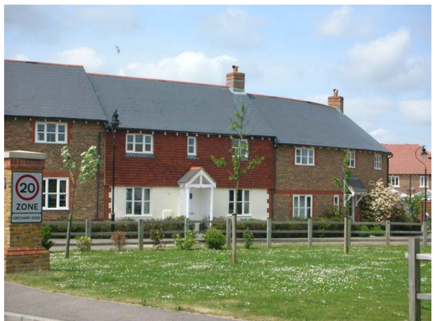
Picture 4.1.3 Good quality design and landscaping
