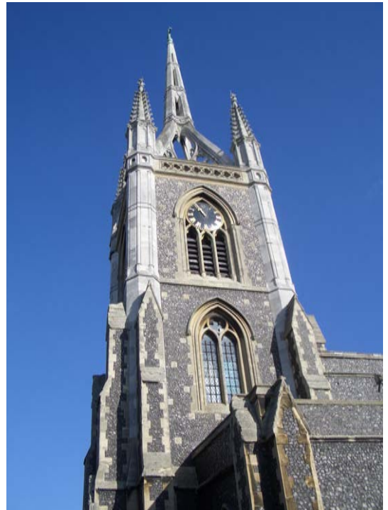
Picture 4.1.6 St. Mary of Charity, parish church of Faversham
